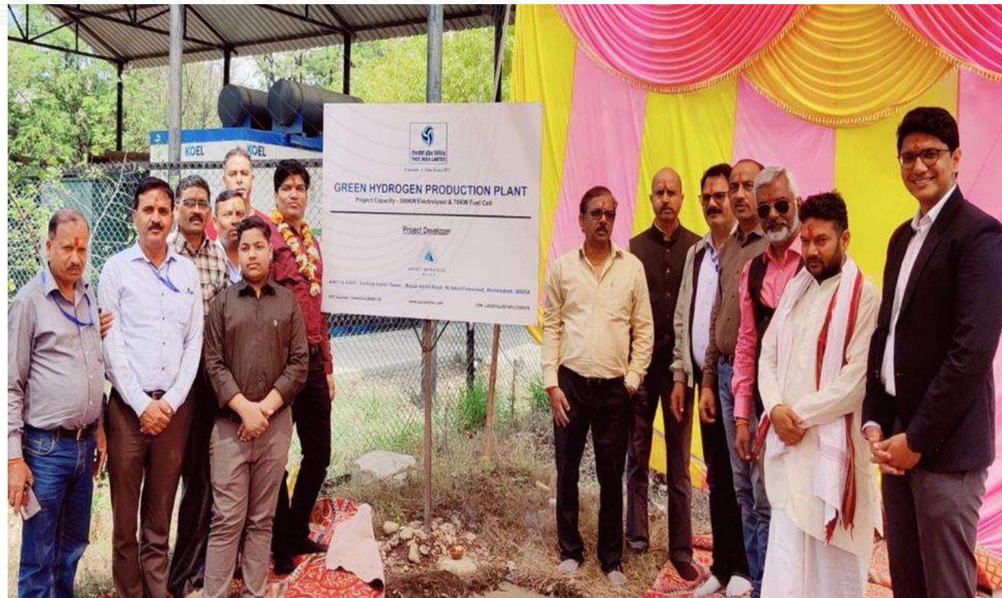
Picture of “ Bhoomi Pujan ” at site in presence of THDC officials and Advait team.
