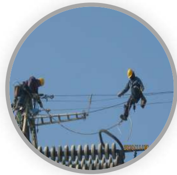
EPC Products for OPGW & Telecom Installation
