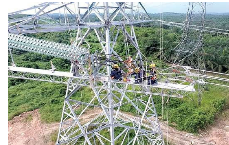
Working Platform (Sag Bridge)
