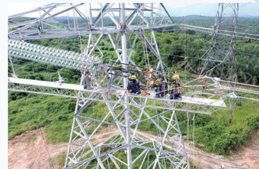
Working Platform (Sag Bridge)
